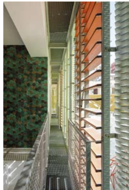
1 Inside metal panels detail
