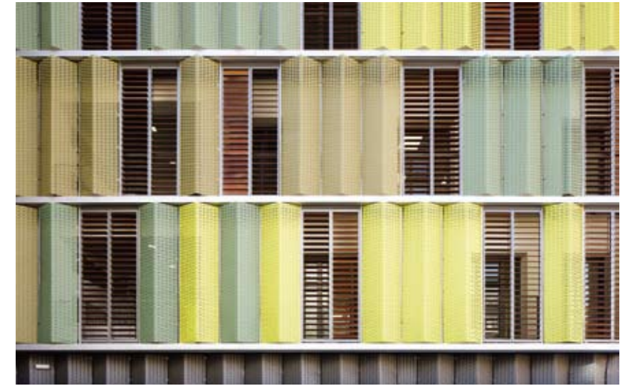
↑ Metal panels facade
